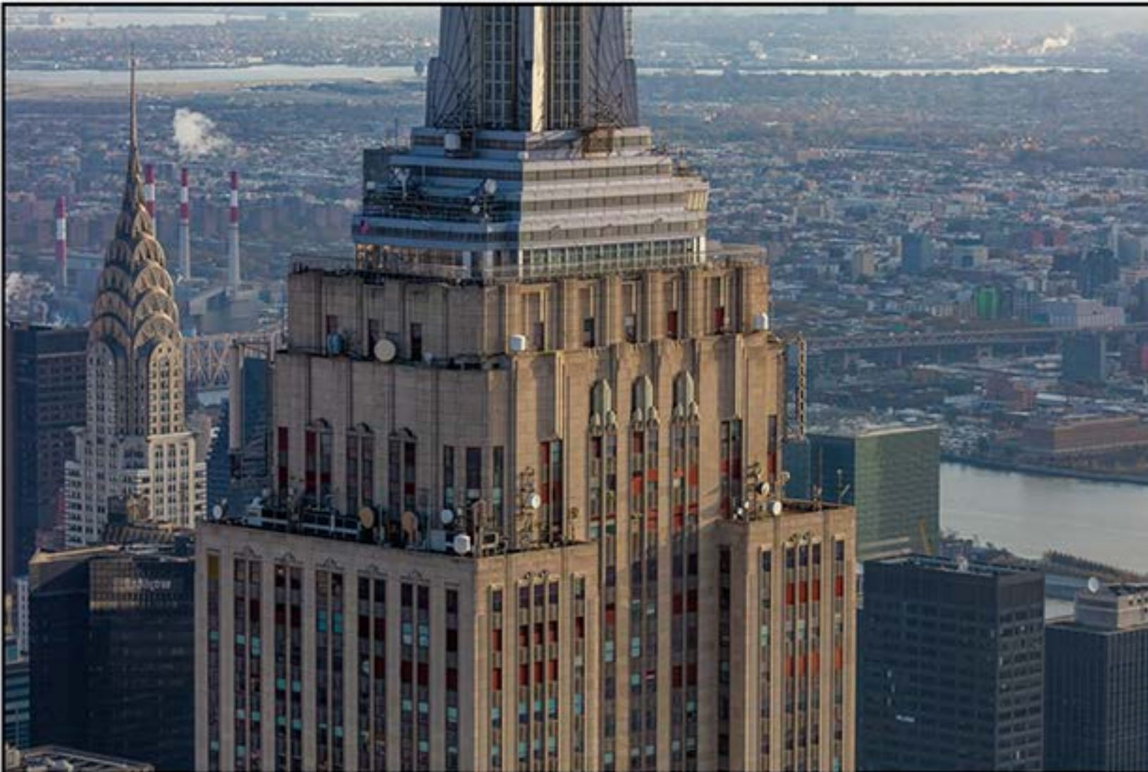
Shreve, Lamb and Harmon, Empire State Building , NYC (1931)
