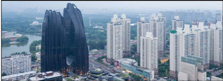
MAD Architects, Chaoyang Park Plaza, Beijing, China (2017)
