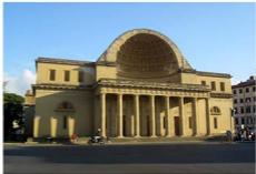
John Outram, Isle of Dogs Pumping Station London, UK (1985 – 88) Right: Francesco Poccianti, Cisternone
