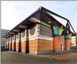
John Outram, Isle of Dogs Pumping Station London, UK (1985 – 88)
